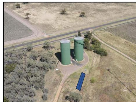
Warren Chlorination Shed
