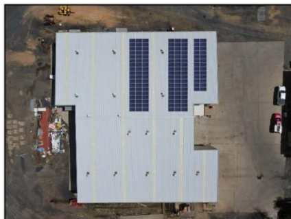
Council Works Depot – 39.5kW
